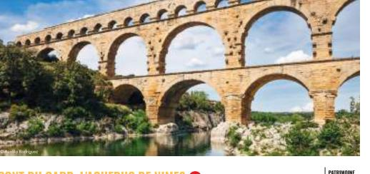
Built in the 1<sup>St</sup> century AD, the Pont du Gard is without a doubt the most spectacular structure of the aqueduct and has been on the Unesco World Heritage List since 1985. The Romans built a bridge of exceptional dimensions to cross the Gardon valley. 275 meters long, 48 meters high (the highest of the Roman world) and three superposed tiers of arches.
